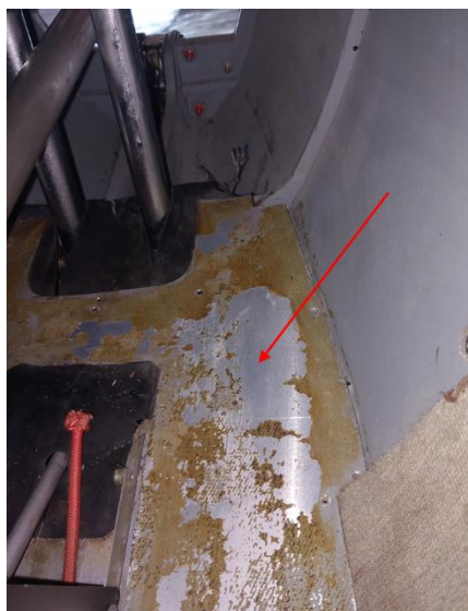
Fig. 4 – Aft section of the cockpit floor
