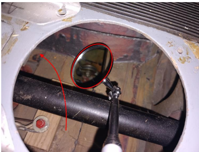
Fig. 10 – Mirror view of the pulley aft of bulkhead No. 3
